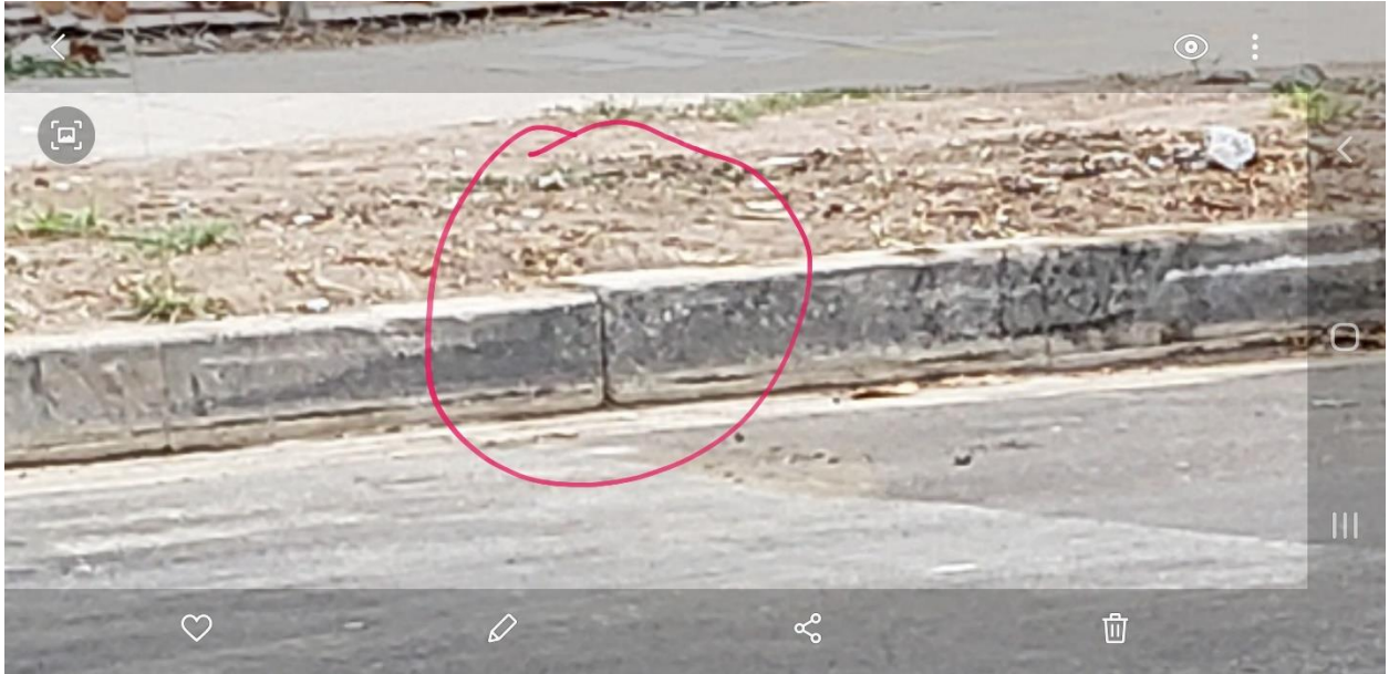
Figure 4 broken curb at fault between CPT 18 and 19
