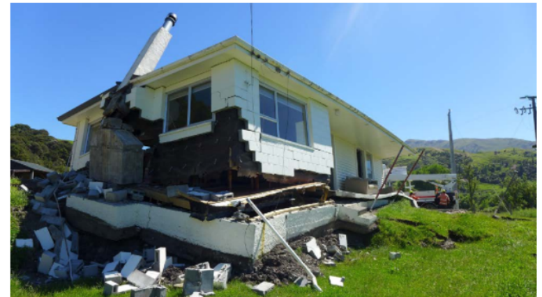
Photo: Cottage destroyed by surface fault rupture on the Kekerengu Fault during the magnitude 7.8 2016 Kaikoura earthquake in New Zealand. Approximately 10 meters of right-lateral fault displacement occurred under this house, tearing it from its foundation. Photo credit: VML 190573, Julian Thomson, GNS Science / Earthquake Commission
