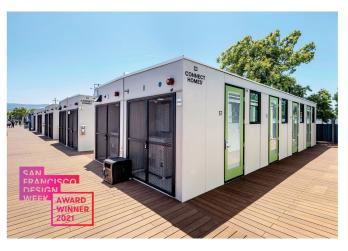
Connect Shelters come in multiple configurations and fire-resisitant wall assemblies mean they can be placed back-to-back and/or stacked for increased density.
