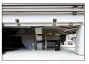
High under module chase space allows for all utilities to run under the crawl space to omit any expensive trenching
