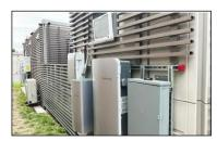
Ability to simply install and run all utility systems through the side wall with single stub-up points for all main utility connections
