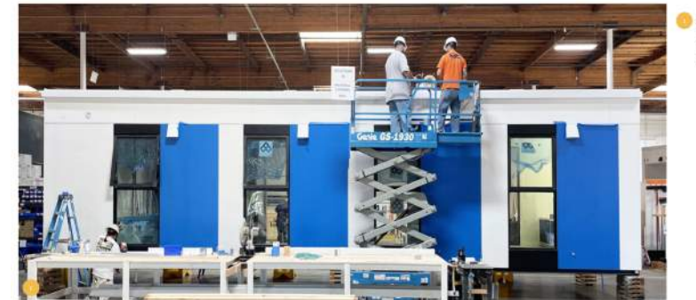
STATION 09: CS-05A: Gutters and interior finishes are being installed at station 9.
