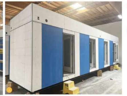
STATION 05: CS-07A: Windows and exterior doors were installed. The module is receiving exterior siding.
